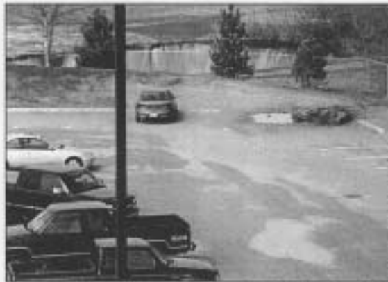
Excessive winter sanding can mean high sediment loading to runoff
